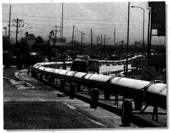
Crews prepare to pull a string of new pipe through a bore under busy 3300 South Street in Salt Lake City. Questar's contractor, Northern Pipeline, used axles and wheels instead of stationary skids to support the pipe. This innovation makes the pipe easier to move and protects the weld joints by not pulling them across the rollers on traditional stationary skids.
