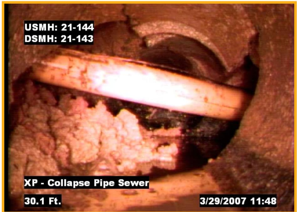
A robotic camera was used to take a picture of this cross bore which is intersection of an existing underground utility by a second utility that compromises the integrity of either utility.
